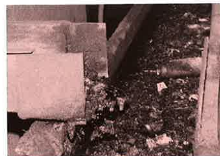
Fig. 64: Wet bottom ash is being conveyed. These units need to be declined at least 2 degrees.
