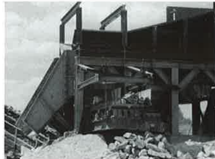
Fig. 45: Large rocks that are called "Rip-Rap" fall down into this conveyor. Its discharge is "picked up" by a loader.
