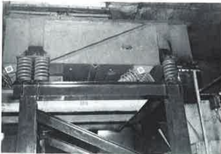
The "short length" feeder under each of the three outlets in line with the belt conveyor. One of them is the center feeder.
