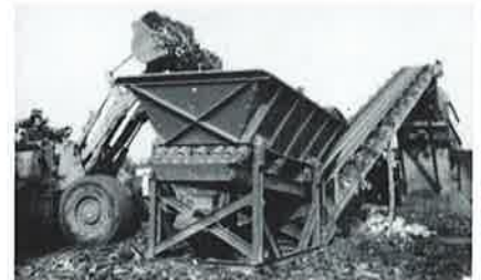
Fig. 39: The "dump hopper" is an integral part of this feeder.
