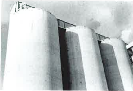
Three 70 ft. diameter by 180 ft. high coal silos.
