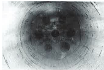
Looking down at the seven outlets in each of the silos. A belt conveyor passes under the three that are horizontally aligned in the picture.
