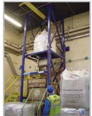
4. Bag loaded ready to discharge.
