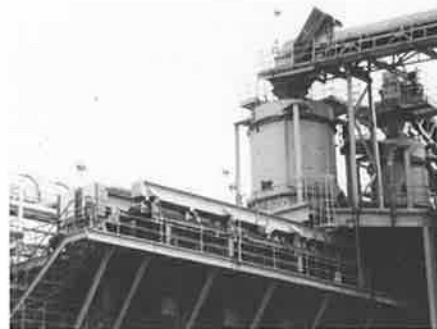
A 1500 cu. ft. - 12 ft. dia. Surge Bin at the upstream end of a Boiler Feed Circuit
